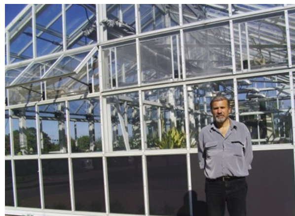
“John Swift, of Solar Tomorrow, shows off the curtain-wall-type solar thermal collectors installed at the research greenhouse at Chatham University in Pittsburgh.”
