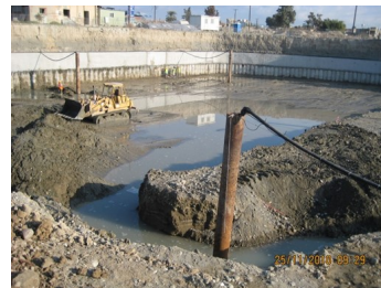
Figure 7 – Construction Stage 5 – Completion of excavation with dewatering
