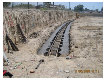
Figure 6 – Construction Stage 4 – Construction of secant pile wall
