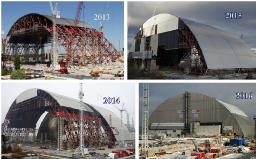
Fig.8: Scientific support for the design and construction of the New Safe Confinement at the Chernobyl nuclear power plant
