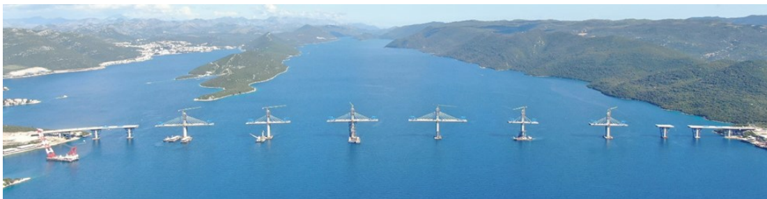
Figure 19. Installation of large segments on approach spans
