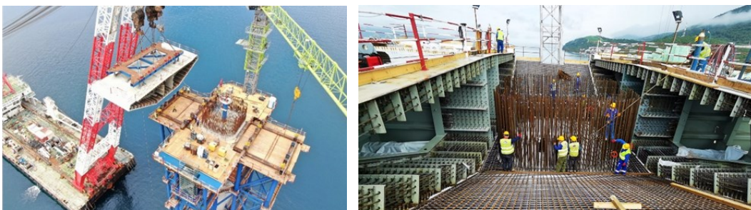
Figure 15. Construction of base segment
