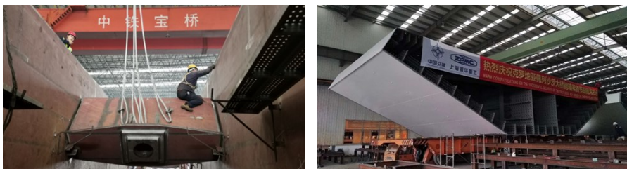
Figure 16. Production of steel segments in production plants in China
