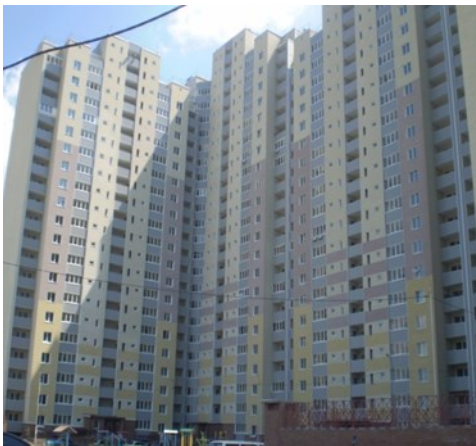
Fig.9: Residential building of the modernized APVS K-134 series with ventilated facade cladding system
