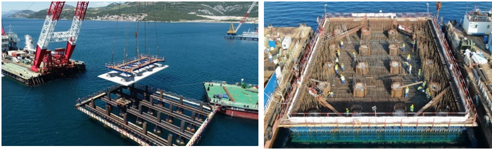
Figure 13. Construction of pile caps
