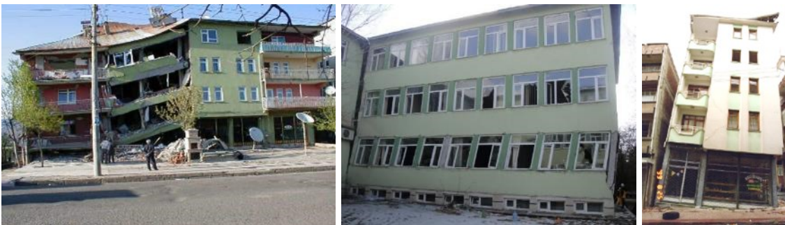
Figure 4. Damaged structures: (a) partial collapse; (b) large residual displacement; (c) rigid rotation
