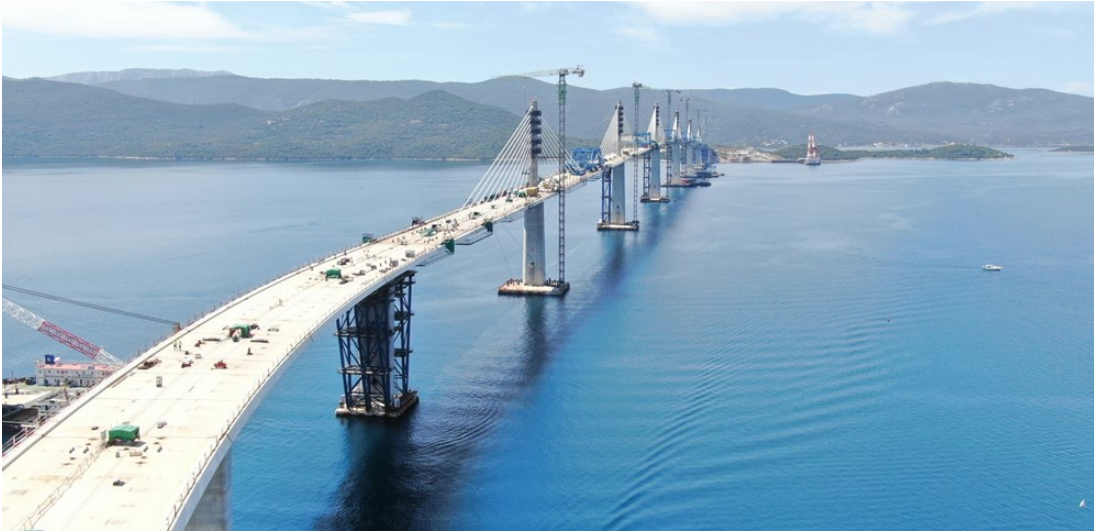
Figure 22. Pelješac bridge during construction
