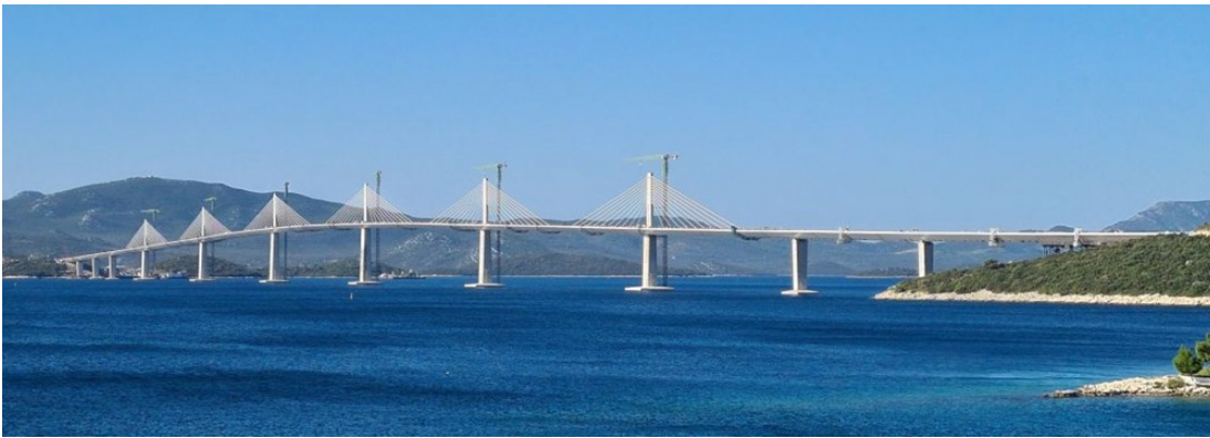
Figure 23. Pelješac bridge, September 2021
