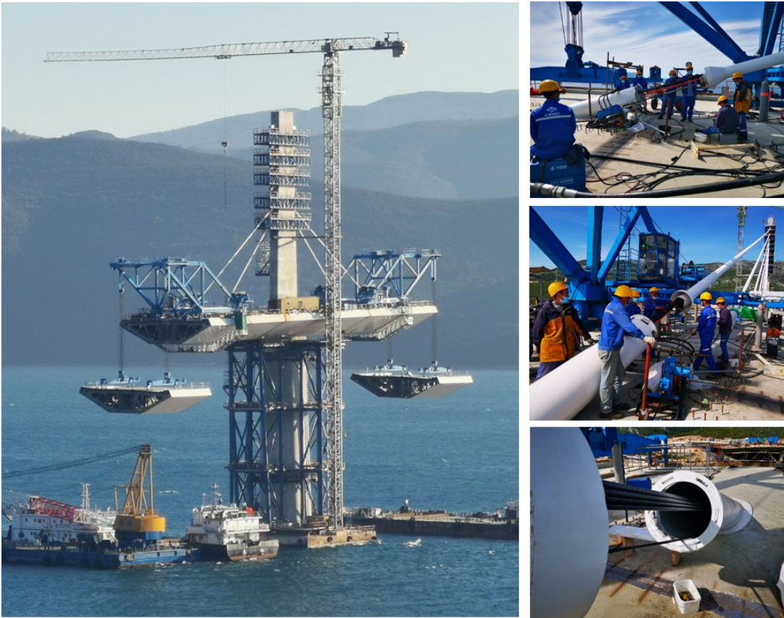
Figure 20. Balanced cantilever construction
