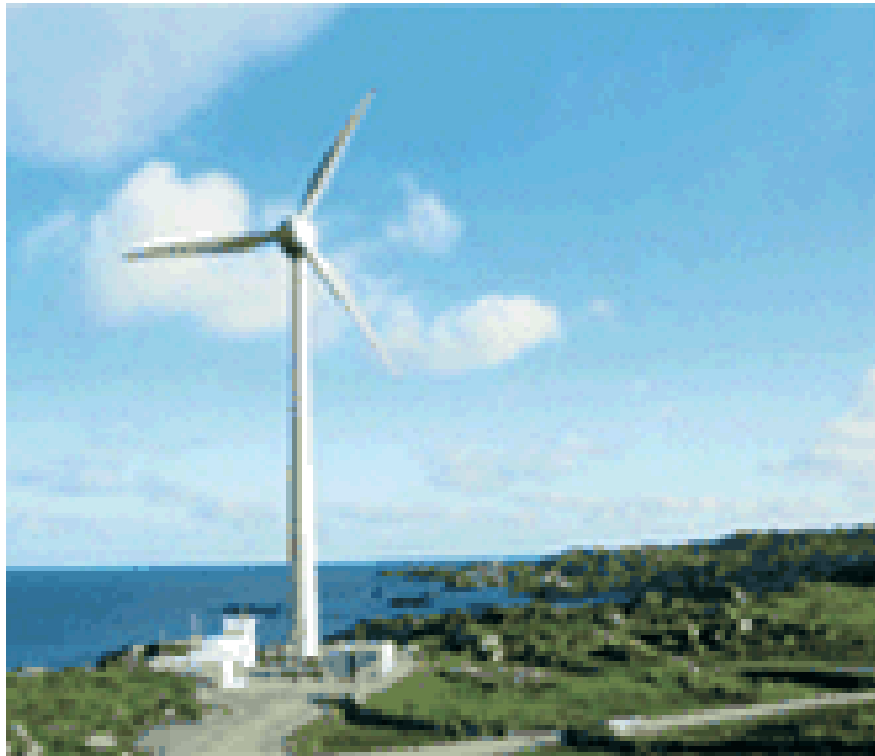
Wind energy plant
