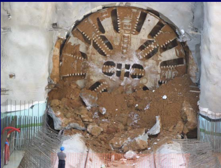
Elliniko station breakthrough
