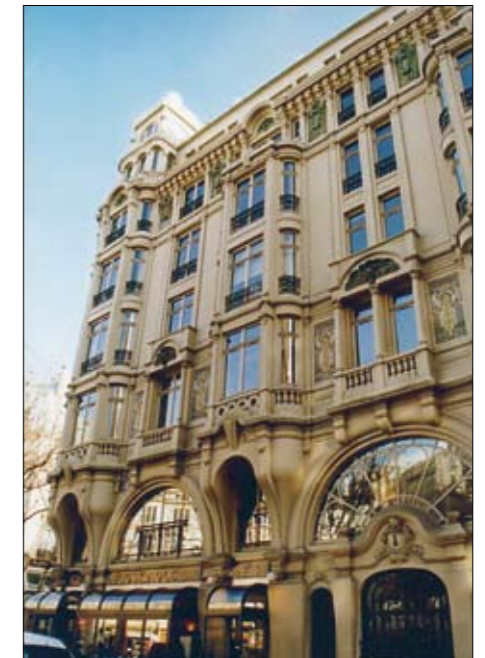
The Hennebique office in Paris was entirely built of reinforced concrete (1901).
