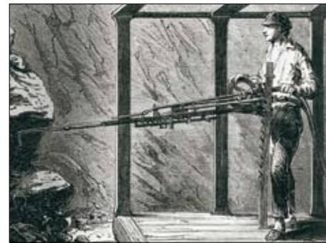
The first pneumatic drilling machine, invented in 1859 by Germain Sommeiller.
