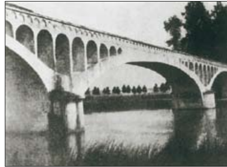
The bridge over the river Yonne in France (built 1870–1873) has the largest non-reinforced concrete arch in the world, with a span of 40 metres. The construction of this bridge was very instructive and had a decisive influence on the further destiny of the first concrete bridges.
