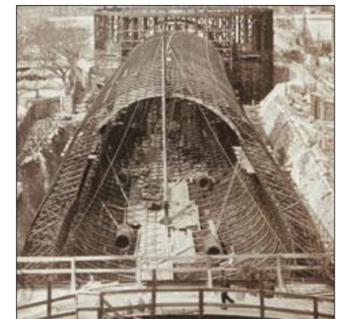
Construction of the Paris metro using iron arches (early 20th century)
