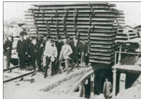
Load test of a concrete arch bridge carried out by Austrian engineers at the end of the 19 th century.
