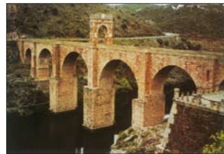
The bridge on the River Tajo at Alcántara in Spain commissioned by the Emperor Trajan in AD 104. It was built by Caius Julius Lacer and has the largest span of any surviving Roman bridge.
