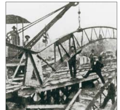
The supporting core of bridges built using the Melan system are iron truss girders.
