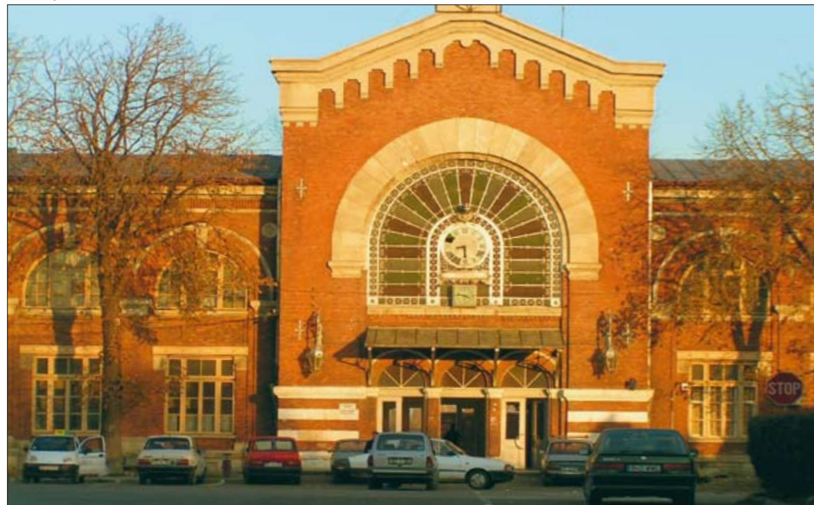
Railway station on the route Buzău - Mărășești line
