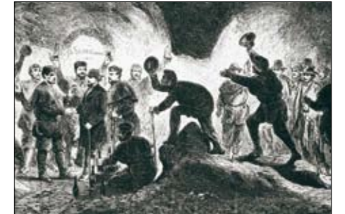
The breakthrough of the Brenner railway tunnel between Austria and Italy; second half of the 19th century.
