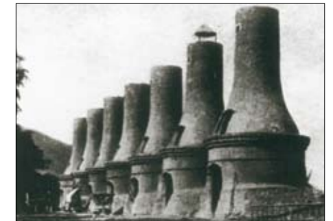
Bottle kiln for the production of cement, built in 1853 by Joseph Vicat (1821–1902) at Gennevrey-de-Vif, France.
