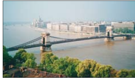
The Chain Bridge in Budapest, Hungary. It was built between 1839 and 1849 and has a central span of 202.6 metres.
