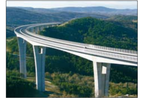
The Črni Kal Viaduct in Slovenia built using the free cantilever method and the Freyssinet post-tensioning system (C-Range).
