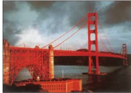
Dr Joseph Melan was the father of the theory of structural behaviour of large suspension bridges. His theoretical research provided a basis for planning and building the largest bridges of this type, including the Golden Gate Bridge in San Francisco. This bridge, built in 1937, held the world record for the longest main span (1280 metres) until 1964. The supporting cables are 90 centimetres in diameter. The Golden Gate is probably the most famous bridge in the world.
