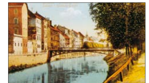
The Shoemakers' Bridge in Ljubljana was one of the first cast-iron bridges in the world to incorporate hinges. It was built in the year 1867 by the Austrian engineer Johann Herman.
