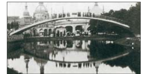
Reinforced concrete arch bridge with a 40-metre span built in 1890 at the exhibition grounds in Bremen, Germany. At its thinnest point the arch measured just 25 cm.
