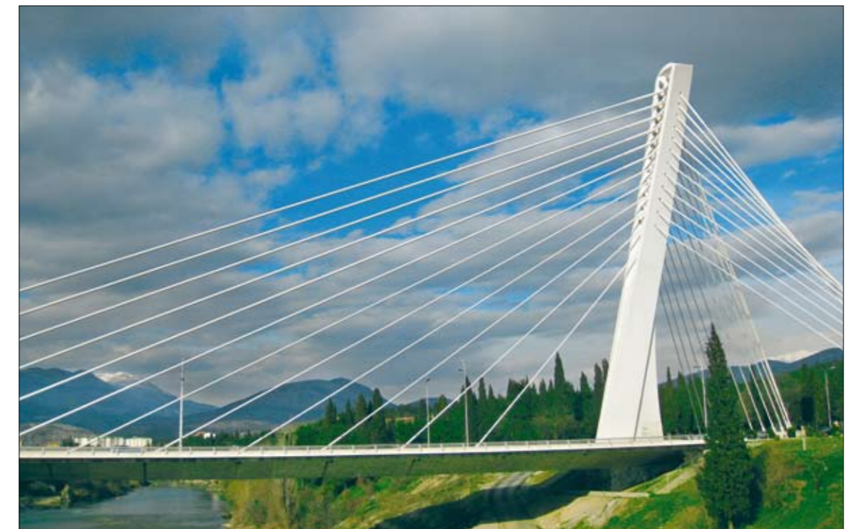
Cable-stayed bridge over the Morača in Podgorica (Montenegro). For the construction of the bridge, which has a main span of 145 metres, Freyssinet post-tensioning and cable stays were used (2004).
