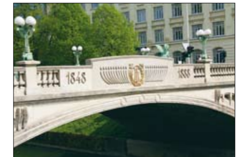
Dragon Bridge - part of the main arch with 3 hinges.
