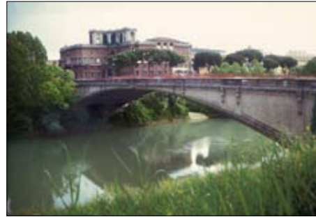
The bridge over the Tiber in Rome was the first reinforced-concrete bridge in the world to reach a span of 100 metres. It was built between 1910 and 1911 by the French engineer François Hennebique.
