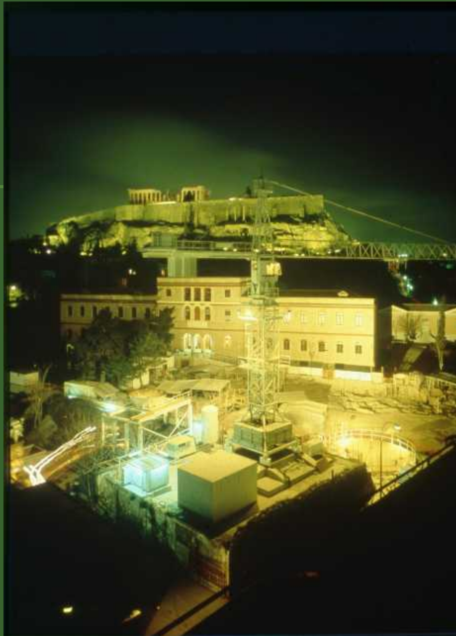
Acropolis Athens Metro Station under construction
